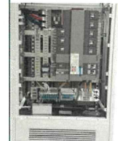
Isolation Transformer & Panelboard
