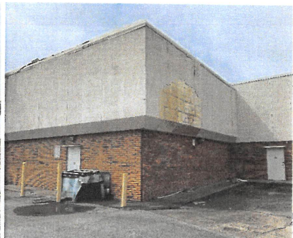
Stagnant standing water near waste collection area; lack of adequate stormwater facilities and drainage
