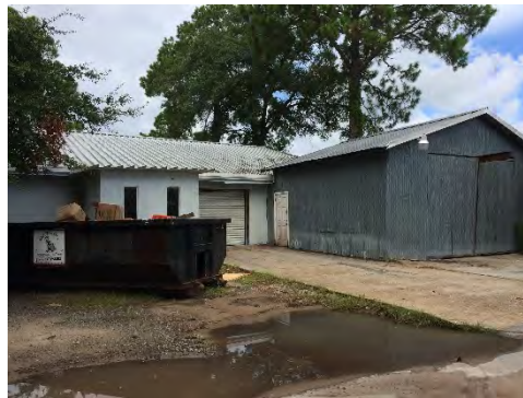
Stagnant standing water, lack of adequate stormwater facilities and drainage
