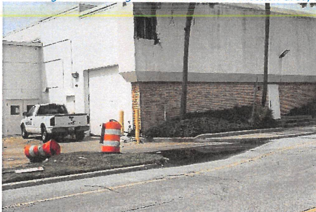
Unsecured building façade, unsecured debris; and structural damage showing the open building envelope.
