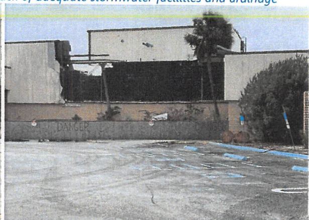
Unsecured building façade, unsecured debris; and structural damage showing the open building envelope.
