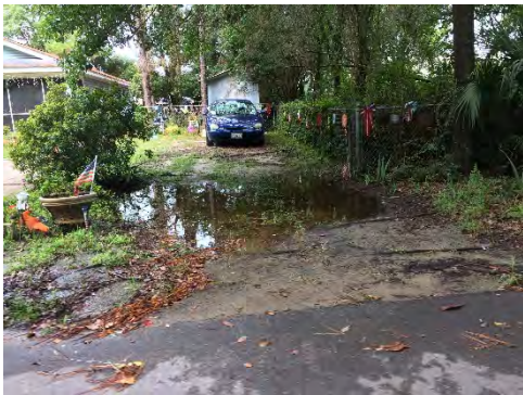
Stagnant standing water, lack of adequate stormwater facilities and drainage
