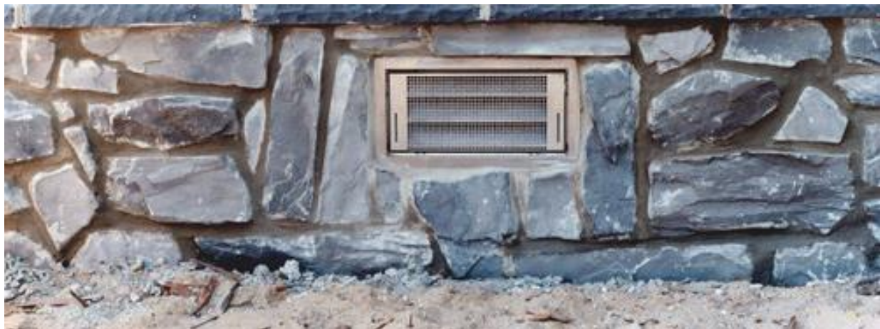
Figure 10. Example of a vent installed on a home to allow wet floodproofing within a crawl space. Source: Floodproofing.com
