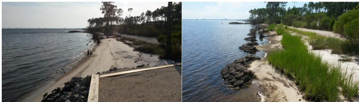
Figure 6. Before (left, 2015) and After (right, 2017) of a breakwater and restoration project using native plant species and recycled oyster shells, completed by students at Deane Bozeman School at RiverCamps on West Bay.
